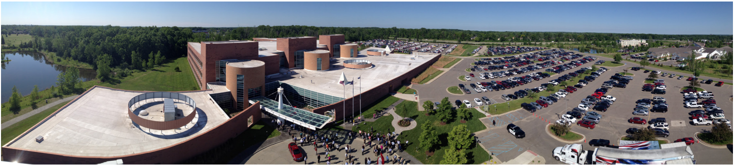
GM Customer Care and Aftersales World Headquarters in Grand Blanc, Michigan
